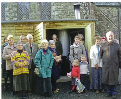
The new boiler house and friends at St Paul's, Gulworthy, Devon
